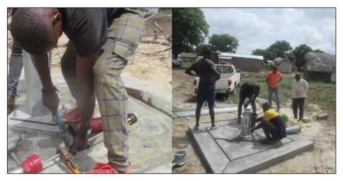
Figure 15: Installation of water well pump mechanism
